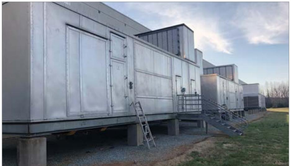
Shown are three AC Corporation Model Z-92000 air washers at the tobacco plant. (Photo courtesy of U.S. Flue-Cured Tobacco Growers, Inc.)
